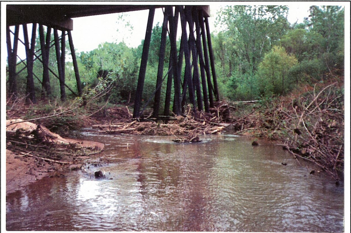
Figure 10. --Debris on pile bent of structure 121007730100 on Interstate 77, crossing Little Rocky Creek in Chester County, South Carolina as viewed from upstream (April 28, 1992).
