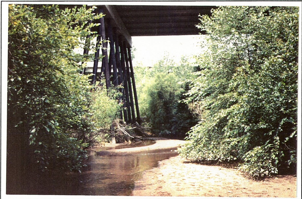
Figure 9. --Debris on pile bent of structure 121007710100 on Interstate 77, crossing Little Rocky Creek in Chester County, South Carolina as viewed from downstream (July 9, 1990).
